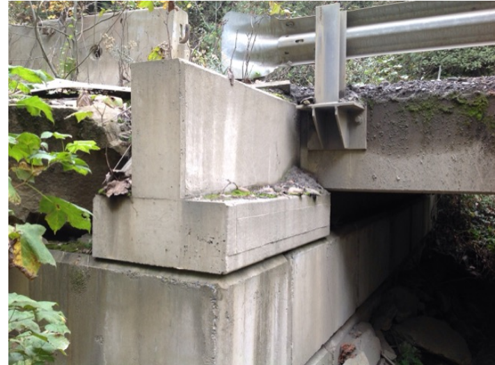
inverted T for ballast wall ends
