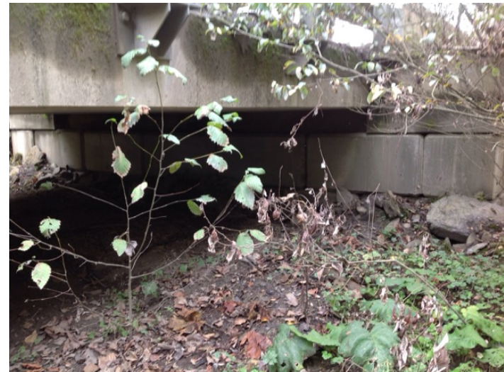
Left Bank Abutment when facing downstream
