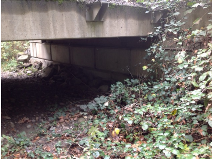
Right Bank Abutment when facing downstream
